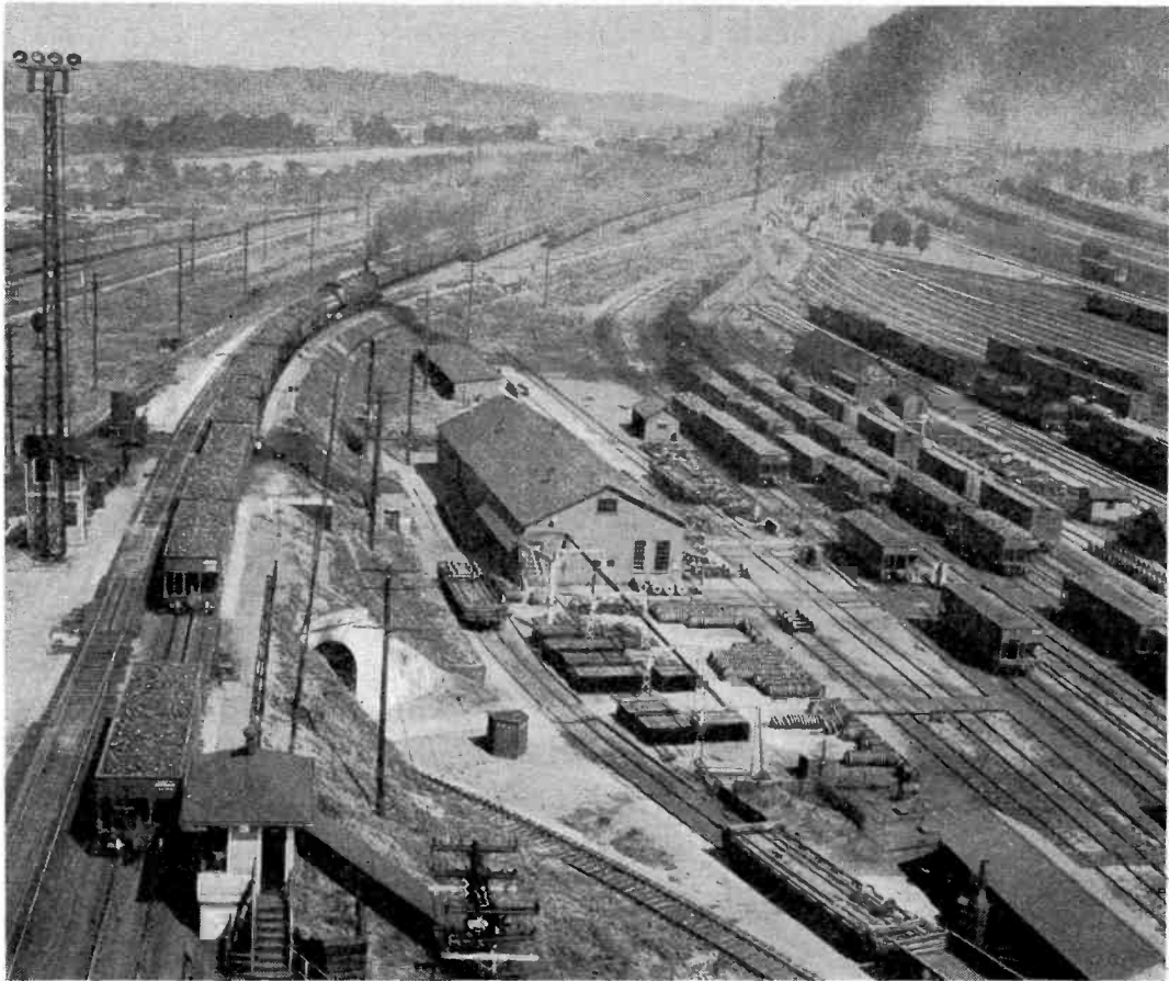
Pictured here is the Westbound Receiving Yard at the Chesapeake and Ohio Railway's Russell Yard in Kentucky. This is one of the largest singly owned and operated railroad yards in the nation.
