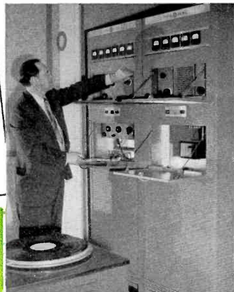
Dwelle S. Hoag, Chief Engineer of W47A, takes readings on the 1-kw FM transmitter
