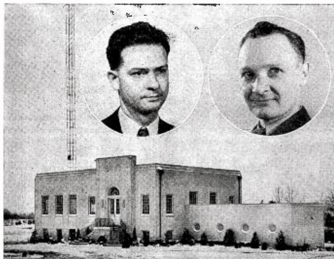
NEW TRANSMITTER PLANT —Of WHAS, Louisville, just completed at a cost of nearly $600,000, of which $265,000 represented latest Western Electric transmitter and speech input equipment and the 654-foot $30,000 Blaw-Knox shunt-excited antenna with beacon. The 50,000-watt outlet is geared to accommodate 500,000 watts, for which WHAS has applied. Insets show Orrin W. Towner (left), technical director, and Joseph Fox, resident engineer. Plant includes modern transmitter house (shown above) costing $40,000, resident engineer's cottage costing $11,000 and caretaker's house costing $4,000, on a tract of 100 acres located at Eastwood, Ky., 19 miles east of Louisville.
