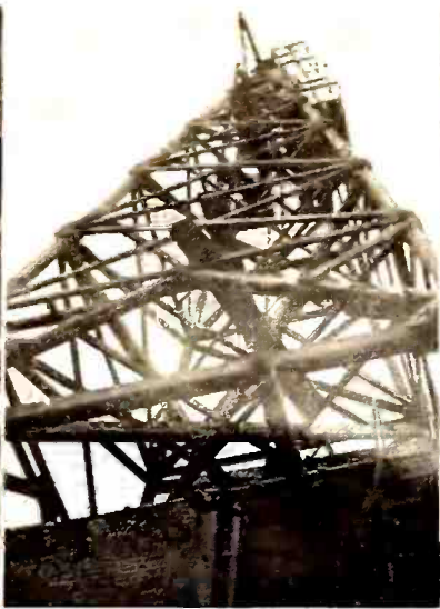
AT PHILCO'S LABORATORIES—At extreme left, Engineer Carl Shumann is working on the "electric eye" tube employed in the television pickup camera. The next picture shows the wooden antenna tower atop Philco's plant in Philadelphia, about 200 feet above ground level, from which the light-to-electricity impulses are broadcast simultaneously with synchronized sound; this tower was struck by lightning recently, caus-
