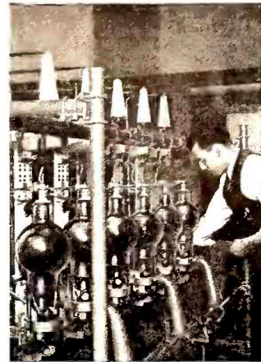
WOR's 17,000 volt rectifier tube unit, with its 6 large Western Electric radiation cooled tubes.
