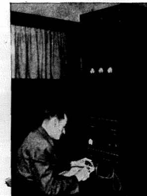
Control Room in New York studio of WINS—showing installation of Western Electric 9 Type Speech Input Equipment.
