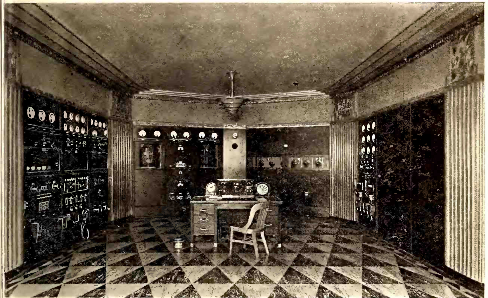
RCA Victor Model 50-B—Fifty Kilowatt Transmitter at WEAF
