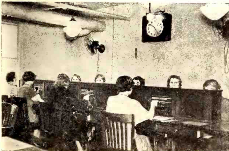
Operators at Special Switchboard of KWK Time Teller Department
