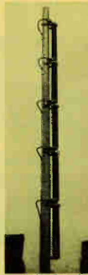
UHF-TV Transmitting Antennas
