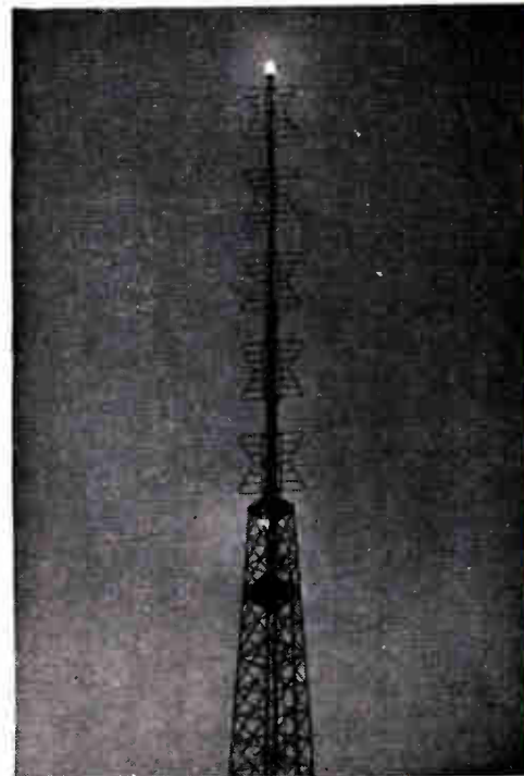
A Television Tower with Crouse-Hinds Obstruction Lighting Equipment
