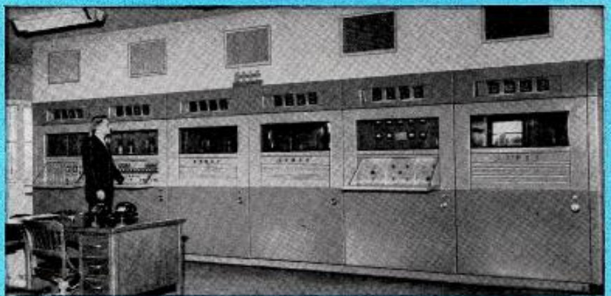
At WDGY, Minneapolis, Minnesota, Mr. K. E. Larson, Transmitter Engineer, trims the RF driver stage of his Westinghouse 50 KW AM transmitter.
