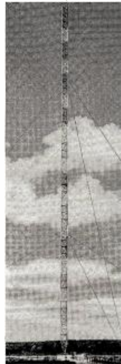
WHDH, Boston, Mass. Three Truscon Guyed Towers; 565 feet, 605 feet, and 645 feet high.
