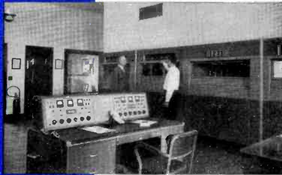
At WHO, Mr. L. A. Sullivan is shown the 50 KW FM transmitter by Station Engineer E. Gfeller. The console controls both the AM and FM transmitters.
