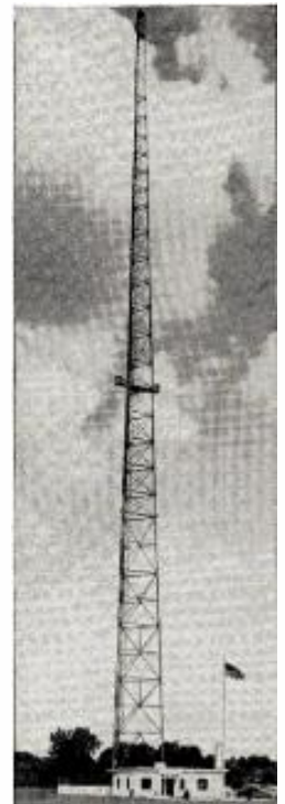
WSAM AM-FM, Soginaw, Michigan, Truscon Self-Supporting Tower, 386 feet high.
