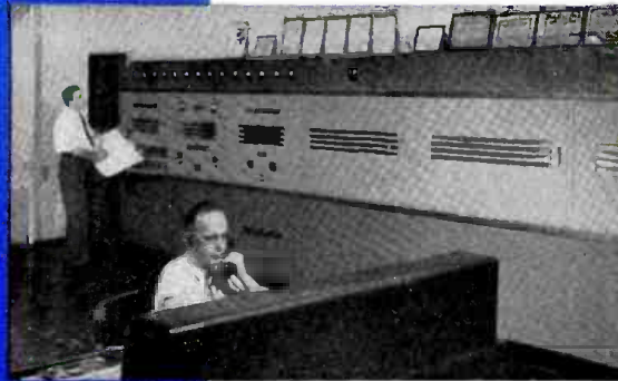
At WWSW, Chief Engineer E. R. Kaiser, standing, and Assistant Chief Engineer J. R. Harlow check their newly-installed Westinghouse 5 KW AM transmitter.
