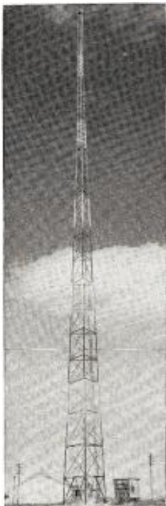
KAA-284, Owatonna, Minnesota, Northern Natural Gas Company, Truscon Self-Supporting Tower, 260 feet high.
