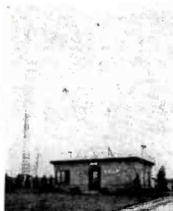
Modern, high efficiency tower.
