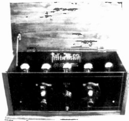
Figure 2. The Long Model F5, a 5-tube TRF with two Kurz-Kasch style dials, with the lid up.
