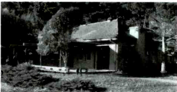
Figure 2. The original radio room building today.
