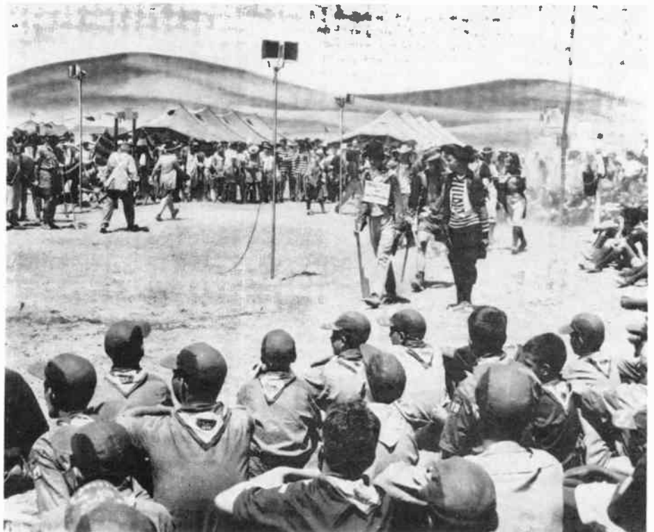
Below: Otto K. Olesen Co. installation of University Cobreflex-2 wide angle speakers for public address system used for Boy Scout Jamboree Week in Irvine, California.
