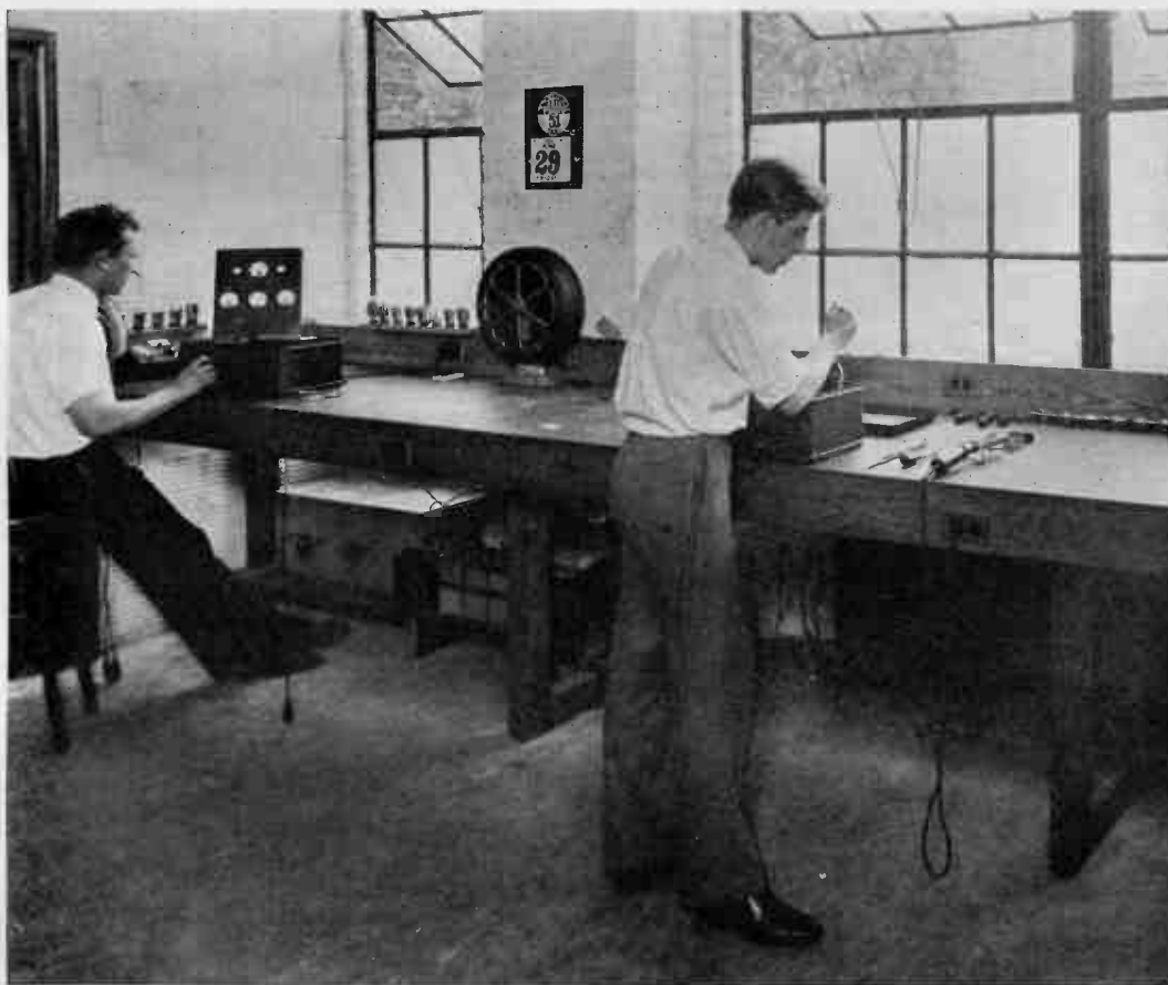
FIG. 34. TWO VIEWS OF A WELL-LAID-OUT SERVICE ROOM.
