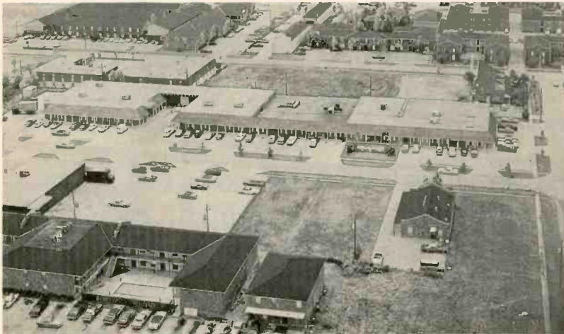
Aerial view of the Swaggart complex
