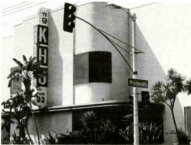
The KHJ building.
