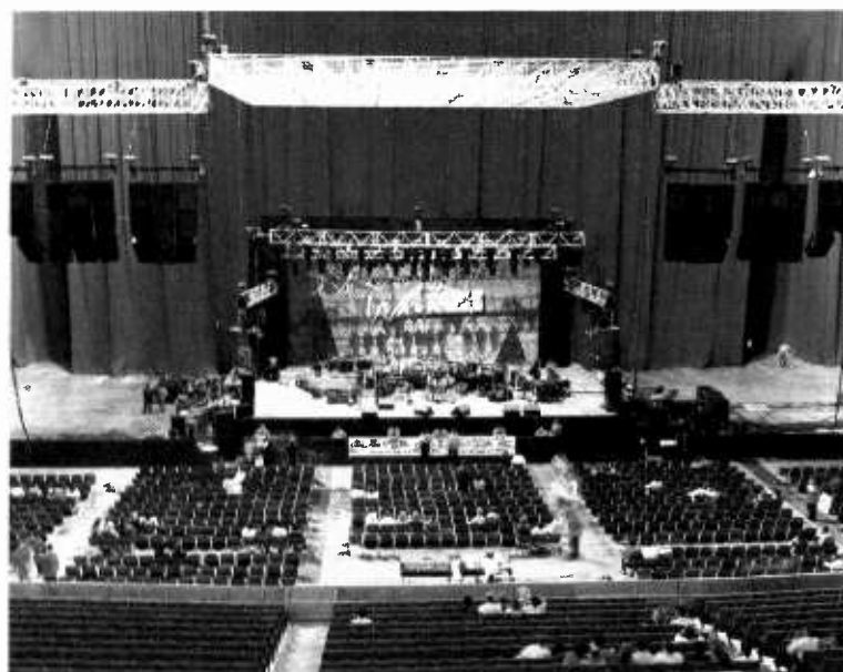
The Louisiana Superdome's new DomeArena features an in-house 40-foot by 60-foot lighting truss and two 8-foot by 40-foot sound trusses.
