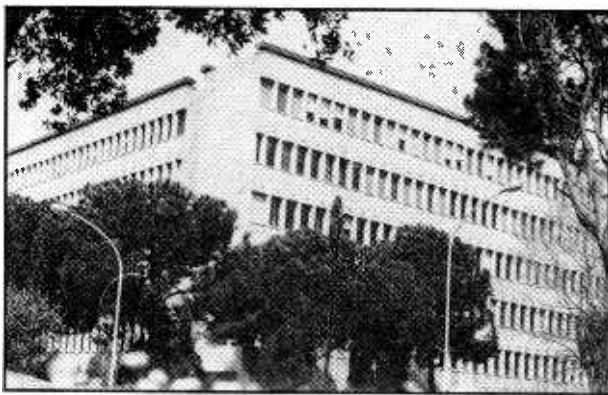
The headquarters of Italian copyright society SIAE in Rome, where more than 700 employees work.
