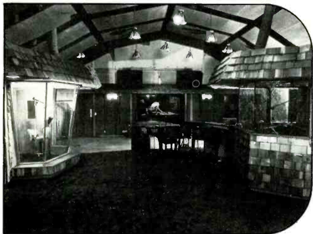
Newly remodeled CBS studio A, with sand-filled floor, low frequency traps, new ceiling acoustics and glass enclosed vocal booth.
