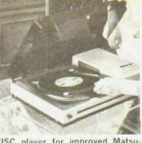
VISC player for improved Matsu shita videodisk system, above, raises upper protective cover at four corners for playback, replacing after USP.
