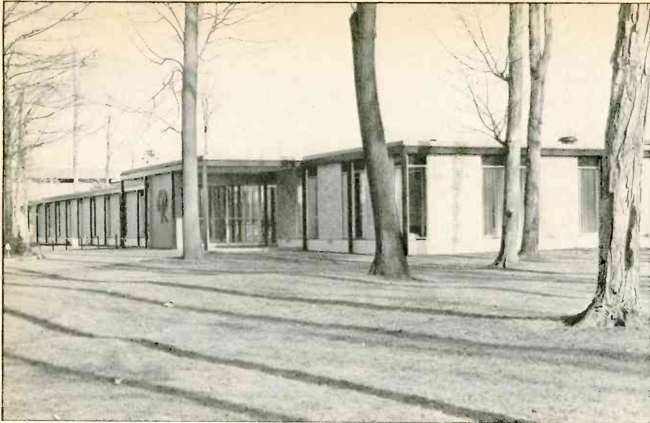
Columbia Records of Canada, Don Mills offices/plant.
