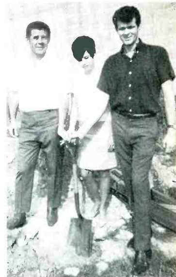
NAT BAILEN, president, Urban Industries, Inc. (left), poses with office manager Patty Mitchell and plant superintendent Don Tyra. The trio was dramatizing the ground-breaking for a new 8,000-square-foot expansion of the Louisville factory, where Panorams are being built.
