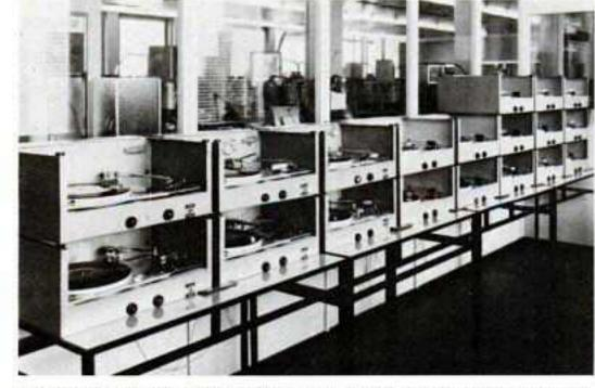
A battery of specially adapted record players in the quality control department of the No. 1 Deutsche Grammophon factory in Hannover. The players are equipped with a second arm which records defects on a slip of paper.
