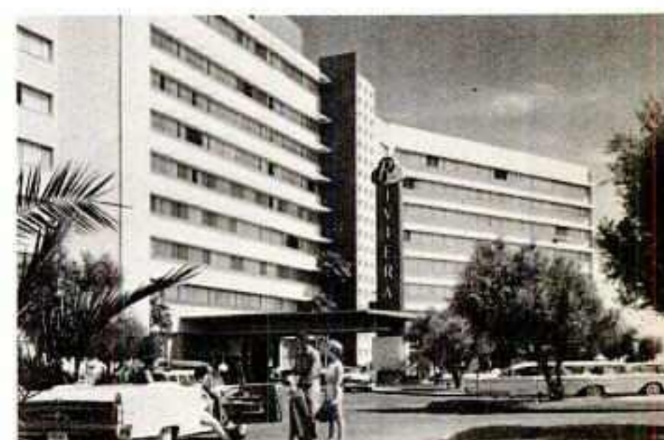
The Riviera's high rise construction welcomes guests to the facility.
