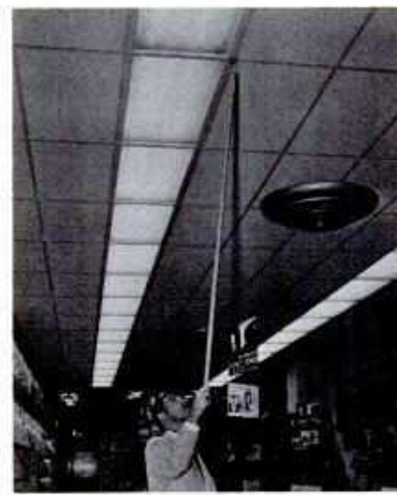
Step Three: Use the pole to stick the hook to the ceiling.
