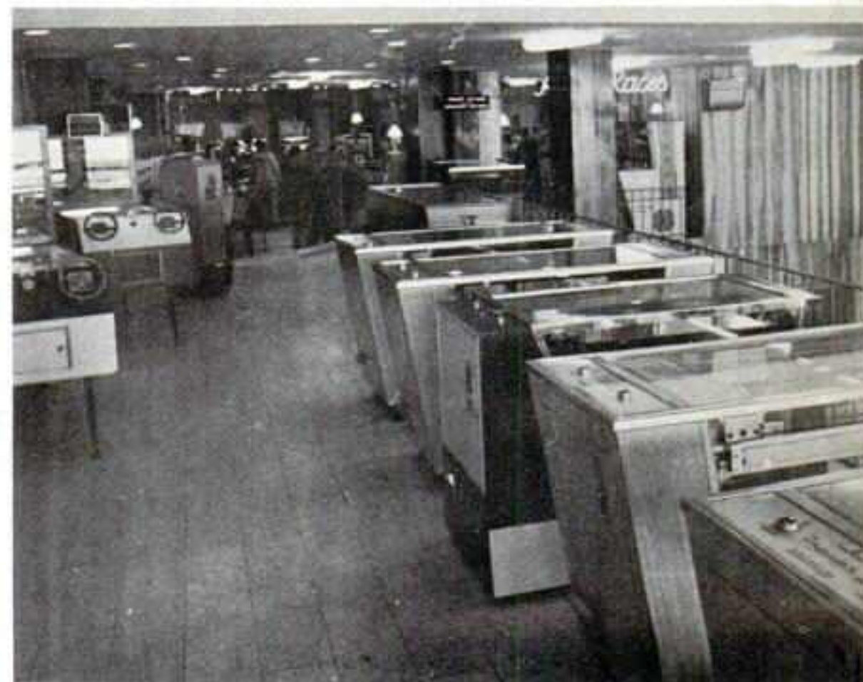
DIGGERS AND GAMES fill the upper floor . . .
