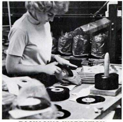
Last inspection: as record goes in sleeve. Spot audio checks are constantly made also.
