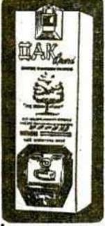
The machine that will bring in extra profits for smart operators is this new Oak Vendor. The machine holds 144 flat pack products. The Oak slip clutch handle is standard The Oak slip clutch handle is standard equipment on each machine. Measuring 26¼" high, 6" wide and 4" deep, this machine will refuse coins when empty and is equipped with an Ace lock and a lock protector. Available with a 25¢ or 50¢ coin mechanism. Wall hinge (pat. pend.) simplifies servicing.
