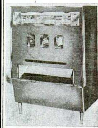
A NEW LINE of Smokeshop cigaret venders, including 18, 27 and 36-column models, were bowed last week. Cabinet has been modernized and several improvements made on the mechanism. Prices can be set from 5 cents to \$1. Selection is electric and capacity ranges from 450 to 850 packs. Eye-level loading and easy swing-out servicing are among the features.
