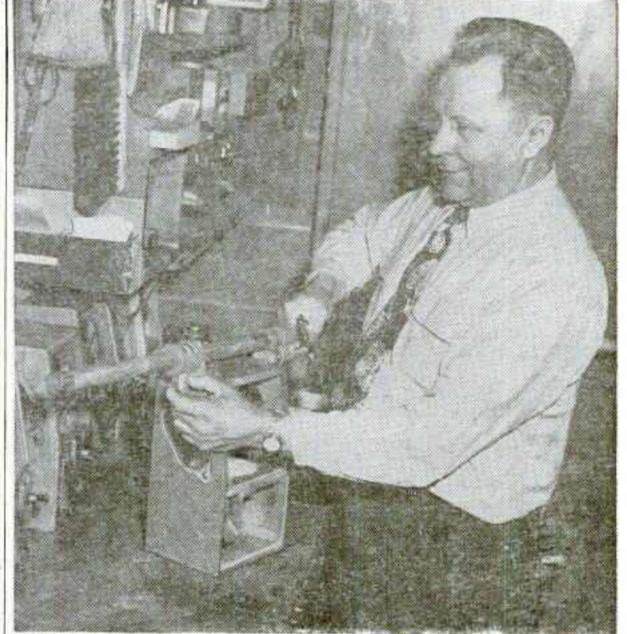
SAMP USES A MANUAL CLAMP TO CEMENT the joints on a rebuilt vending machine for his route. His immaculate machines and sparkling maintenance program are a trademark.
