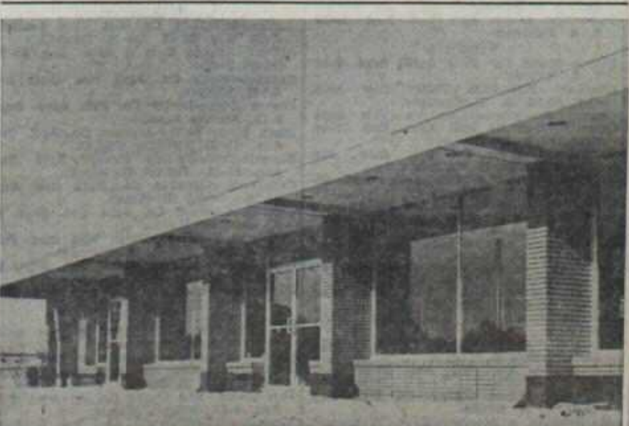
A modern eat-and-drink set-up is the above $135,000 refreshment building at the new Westbury (L. I.) Drive-In Theater. Features include direct concession-to-car service by attractive car-hops and a large outdoor terrace for dining service while viewing the movies. Choice of food includes pizza, hot dogs, shrimp rolls and hamburgers.
