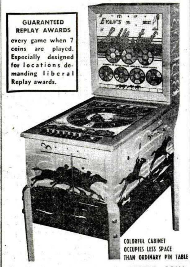
Greatly improved new style SINGLE COIN DROP (WITH SLUG REJECTOR) easily accessible on push-button plate. 5c or 10c play. High scores possible with single coin for top-play incentive.
