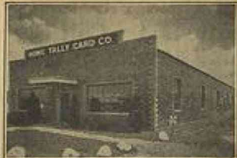
NEW PLANT of the Home Tally Card Company, one mile east of Yorktown, Ind., built to take care of expanding business. The two-story structure has 5,000 square feet of space.
