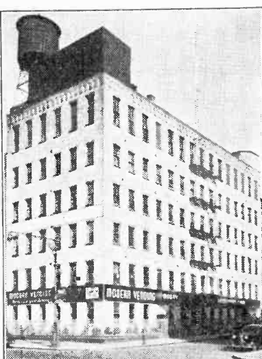
MODERN VENDING COMPANY'S uptown offices in the center of New York's Coin Machine Row. The building was formerly occupied by East Coast Phonograph Company. Modern has redecorated and refurbished the entire building, in which it maintains a complete display of Seeburg phonographs and music systems.
