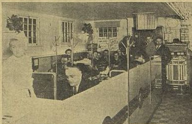
SEEBURG WIRELESS REMOTE CONTROL music system was recently installed in this coffee shop in Mead, Ill. Location is reported to have noted increased popularity since installation. This is a complete wireless remote control installation in one of the smallest of locations.
