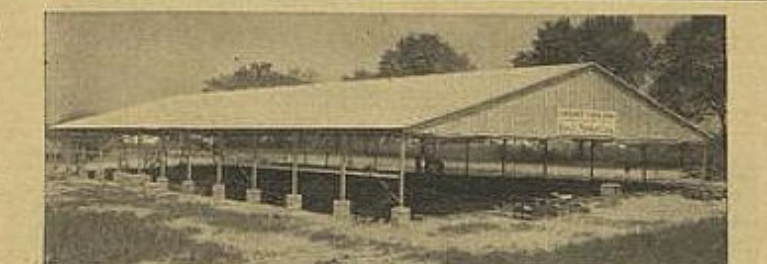
SAID to be an innovation in portable rinks is the new all-steel 60-by-120-foot Tri-State Roller Rink, illustrated above, which opened recently near Evansville, Ind., under proprietorship of William Barton. J. C. Boydston is floor manager. Furnished by George L. Meeker Co., framework and pressed roof sheets are of galvanized steel. Budding may be erected or dismantled with ease, as parts are numbered.
