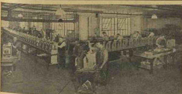
BILLS' FAMOUS BELL LINE is shown above, with workmen busily fitting the machines for waiting operators. The chap in the black suit, left of center, is Joe Luba, foreman of the department.
