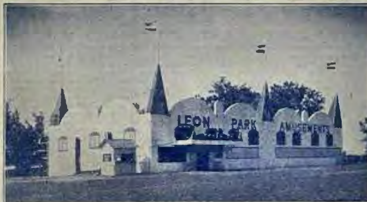
MAIN BUILDING IN LEON PARK , Miles City, Mont., where this amusement spot, situated on banks of the Yellowstone River, "was started from a cow pasture," say D. P. and L. E. Leon, brothers, who are the operators. For several years the playland has been gradually developed and management is anticipating a good season, with dance bands and free acts featured and augmented equipment in its Sportland.
