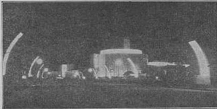
A NOVEL LIGHTING EFFECT FOR WALKWAYS is produced by these indirect pylons. Reflecting surfaces are lit by floodlights concealed in base. An additional effect is produced by exposed sources.
