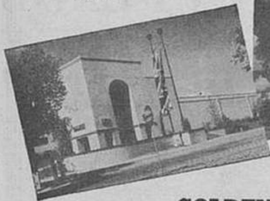
Poultry Building .. 30,000 square feet of space
