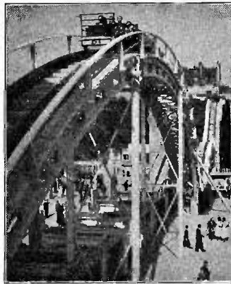
CYCLONE COASTER, operated by Harry G. Traver, American ride builder, with Leonard Thompson, Blackpool, England, in the amusement park of Paris International Exposition, is known as the fastest gravity coaster in Europe. Total length is 3,000 feet and height of first of the 11 dips is 67 feet. Arch of the Coaster, 140 feet wide, is used as main entrance to the park in the heart of Paris in the Esplanades des Invalides.
