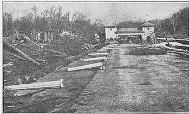
CONCRETE LIGHT POLES WERE LEVELED during the January Ohio River flood, which inundated Coney Island, Cincinnati, to a depth of 25 feet. This view looks out of the park toward the main entrance and shows roads and lawns covered with driftwood and other debris. Some of the white sand of the swimming pool is seen on the right, altho the front pool building is missing.
