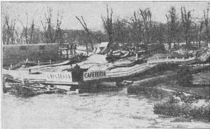
WRECKAGE OF THE BIG CAFETERIA at Coney Island, Cincinnati, was strewn about the park during the recent flood. Photo shows part of the roof and the two signs swept from original location and resting upon a concrete walk near the mall. Numerous strange buildings were washed downstream and deposited against trees and ride structures.
