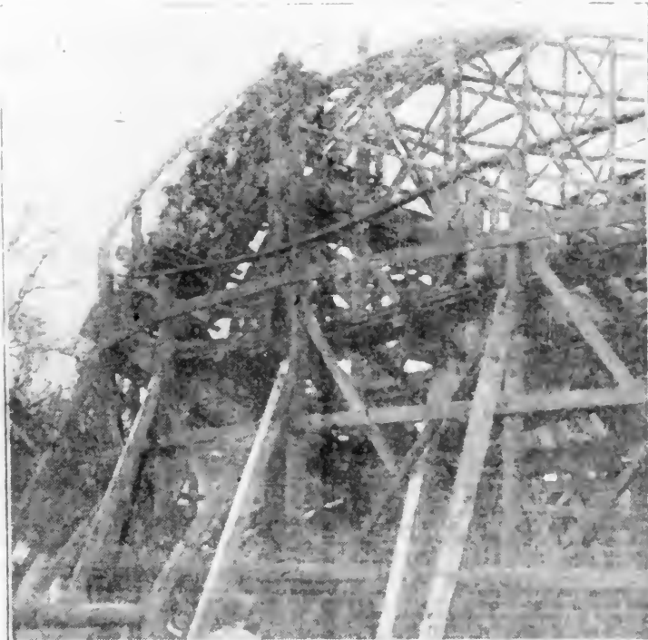
Reproductions of the famous new "Bobs" coaster Riverview Park, Chicago. It was designed by Fred Church and built by the Traver Engineering Company, of Beaver Falls, Pa. The dips are all on steep, spiral curves, banked up to 45 degrees. Only the patented flexible train can be used on these special dips.
