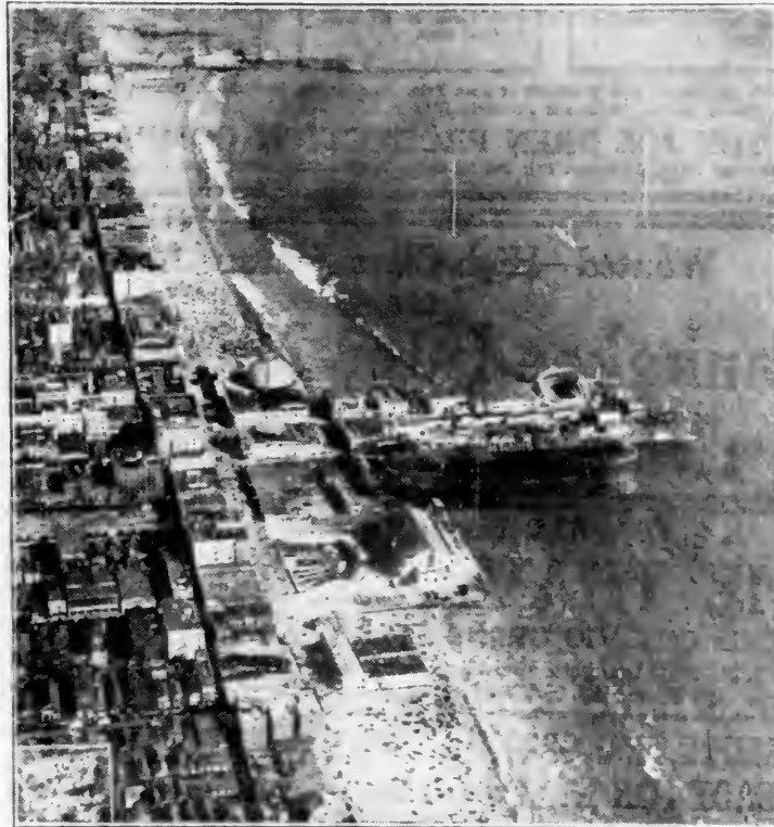
Herewith is seen the amusement zone of Ocean Park, Calif., as it appeared before January 6, when fire destroyed practically all buildings, rides and attractions, causing loss of more than $1,000,000. Near the water's edge, in the foreground, is the bath house, formerly owned by the L. A. Thompson Scenic Railway Company, of New York, thru whose courtesy this splendid aerial photograph, taken by Wm. L. Cross, of Los Angeles, is reprinted. Next is the municipal auditorium and bandstand and other properties up to Lick's Dome Pier.
