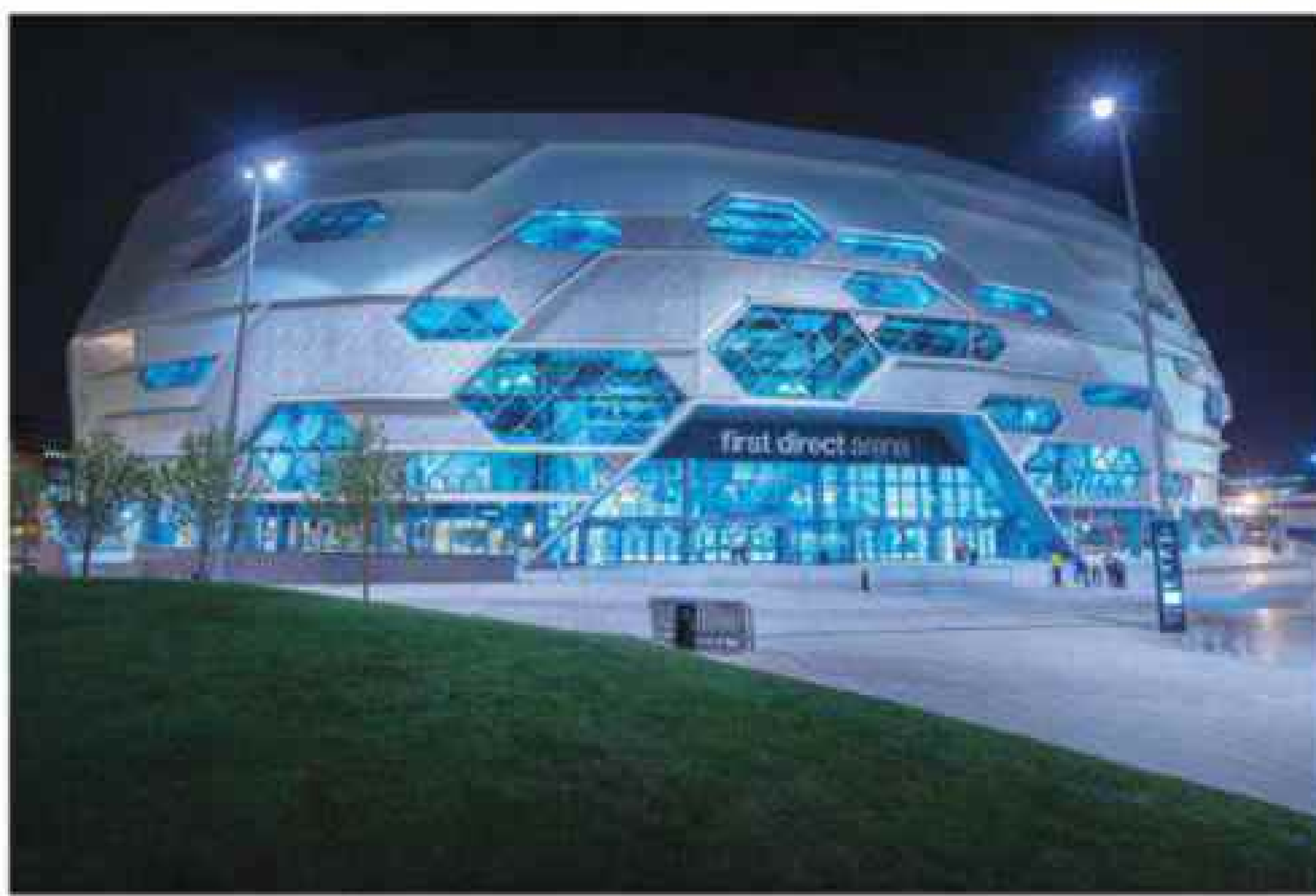
The exterior of the First Direct Arena in Leeds, England, can be custom-lit for different events.
