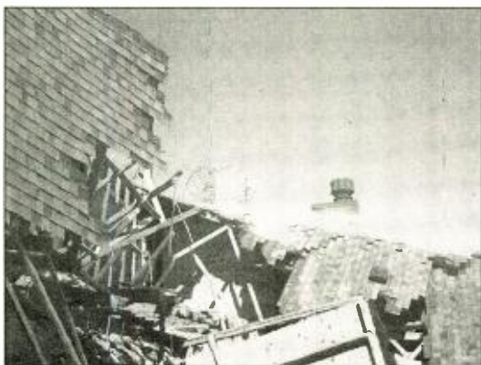
BRINGING THE OUTDOORS IN Sure, 30 inches of snow may sound fabulous — if you're climbing Mt. Everest, maybe. Not so great if it's concentrated on the roof of, say, a radio station in Denver. Here's an up-close look at the building that houses KOSI, the morning after the roof caved in.
