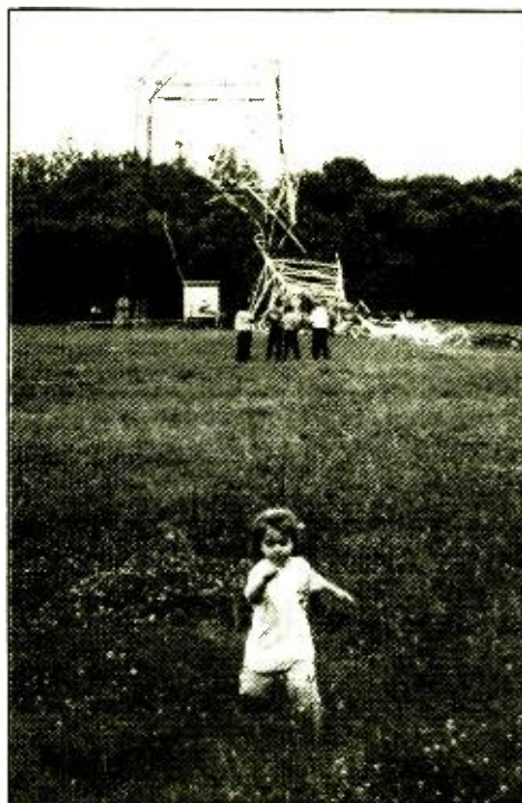
TODDLER TOPPLES TOWER — Carly Bender, daughter of WNDE & WFBQ/Indy OM Marty Bender, looks mighty suspicious running away from WNDE's recently tumbled tower. The mystery of the tower's fall has — officially — not yet been solved.
