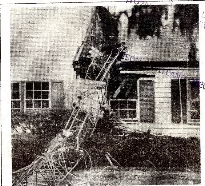
I FALL TO PIECES — For the third time in the last ten years, WKOX/Framingham-Boston has seen its tower topple. The new stick, built for WKOX's recently-granted nighttime power, split the station's studios and landed in the parking lot. WKOX was only one of Hurricane Gloria's victims, as the storm also destroyed WBLI/Long Island's tower and wreaked technical havoc on scores of stations along the Atlantic coast. Photo courtesy of the Middlesex News .
