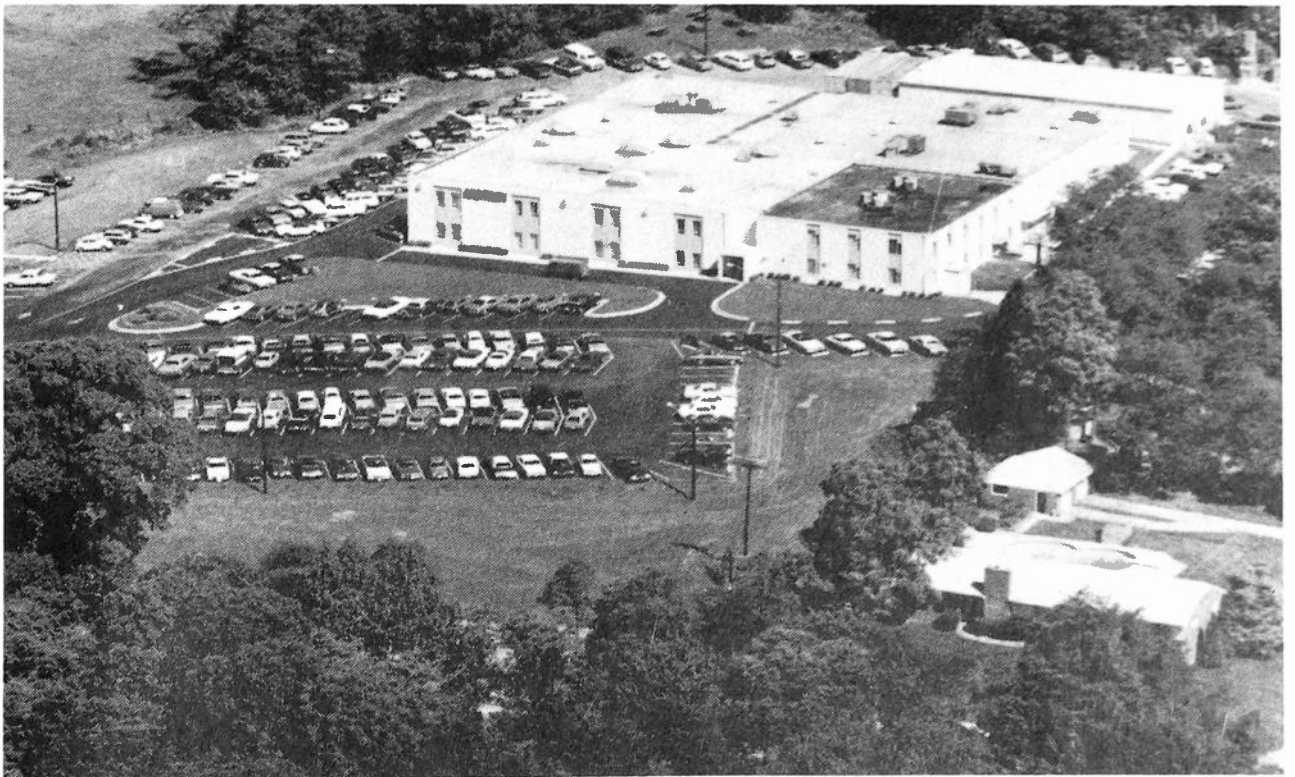
Aerial view of Arbitron Headquarters, Beltsville, Md.
