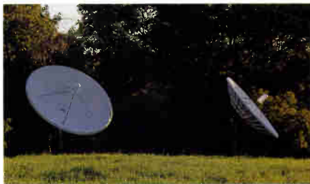
At TV 43, primary programming is received on a fixed Microdyne antenna. The VistaLink antenna rotates to receive programming from other satellites.
