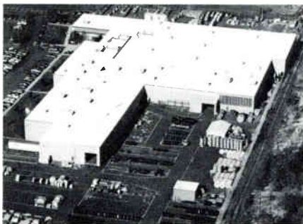
Cablewave's North Haven, CT plant.
